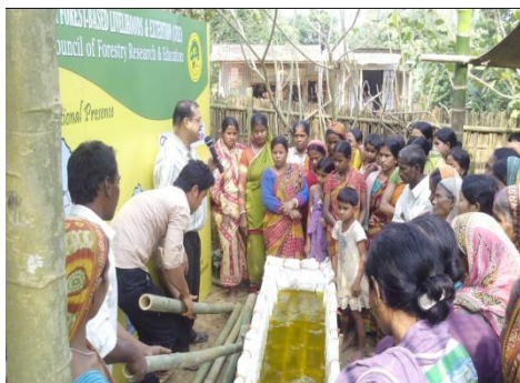
Bamboo made Treatment Tank at Noagaon
