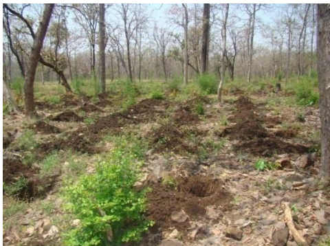
Pit Digging at site
