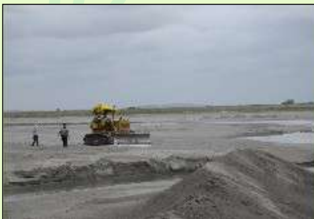
An active fly ash dyke in SSTPP
