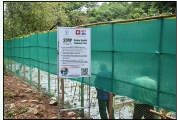
Fencing with bamboo poles + agro net + plastic wire mesh
