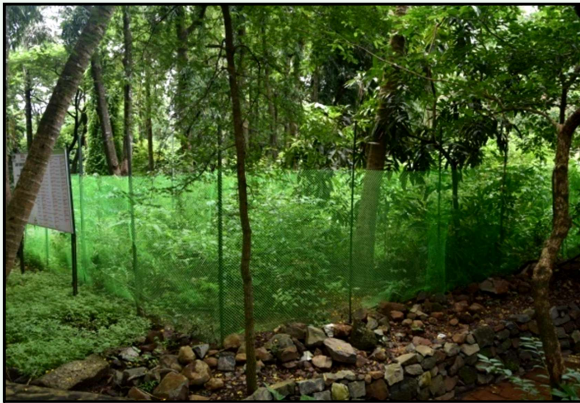
Fencing with plastic wire mesh with iron pole
